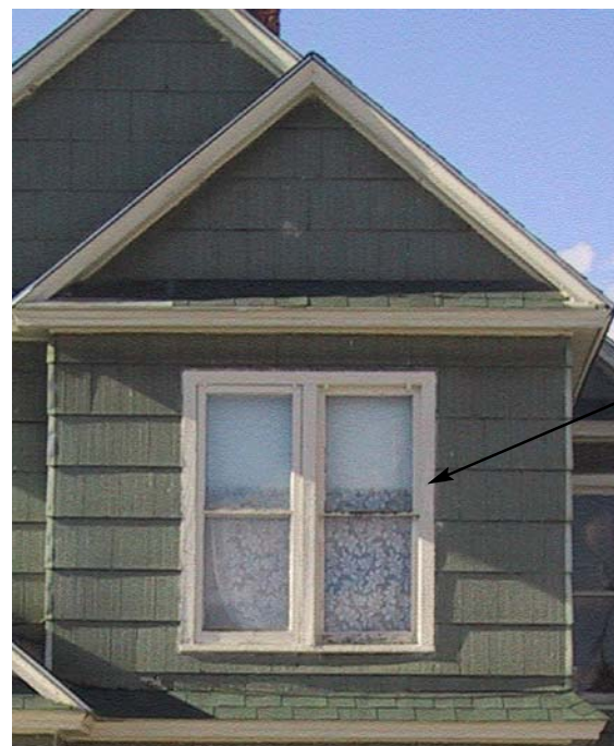
Wood Construction: trim on four sides
