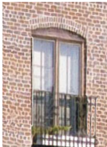
Brick segmental arch
